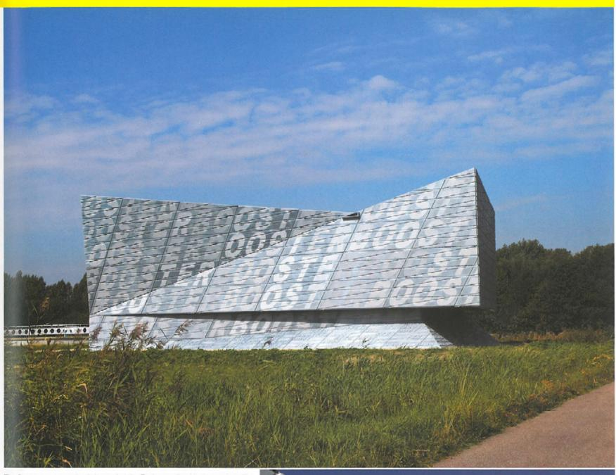
The Booster pump station is located at the Zeeburgereiland in Amsterdam. The building accommodates three Booster pumps. All the sewage of Amsterdam East will be collected by these pumps and pumped through to the new central sewage purification centre in Amsterdam West.
