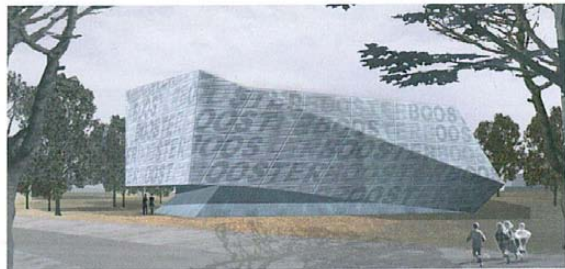
02. Booster Pumpstation Juliette Bekkering Architecten DWR Ingenieursbureau (SE)
